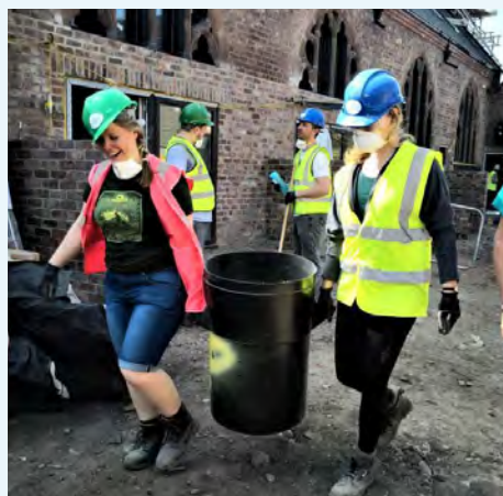
HP Sonia Chapman and Volunteer Rachael Hickmott working on site
